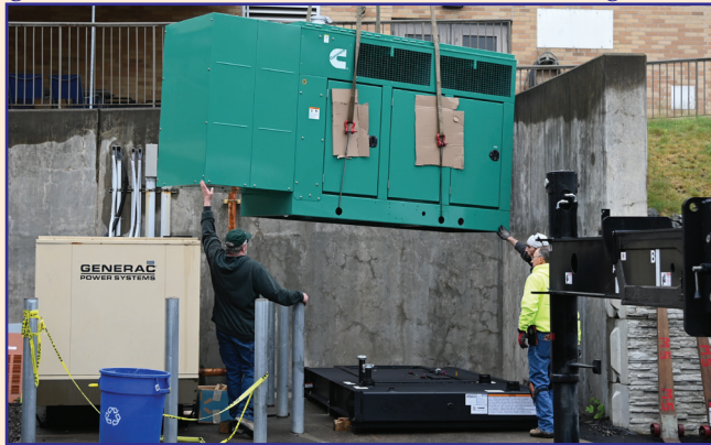
The brand new generator gets installed at the Main Center.
